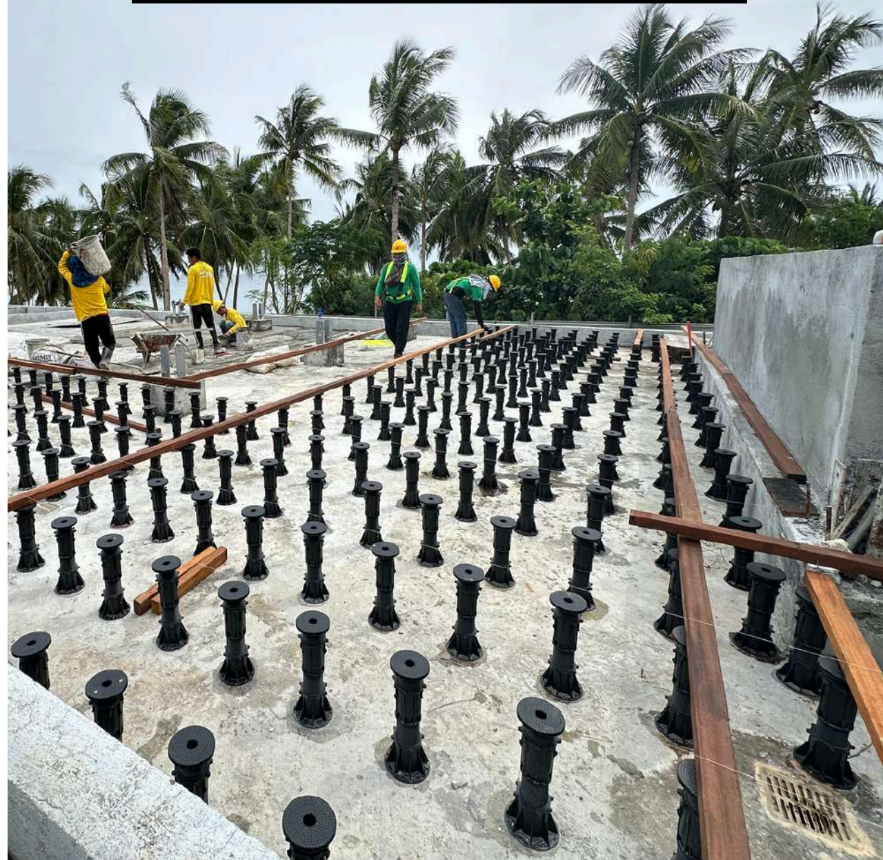
INSTALLATION USING PEDESTAL
