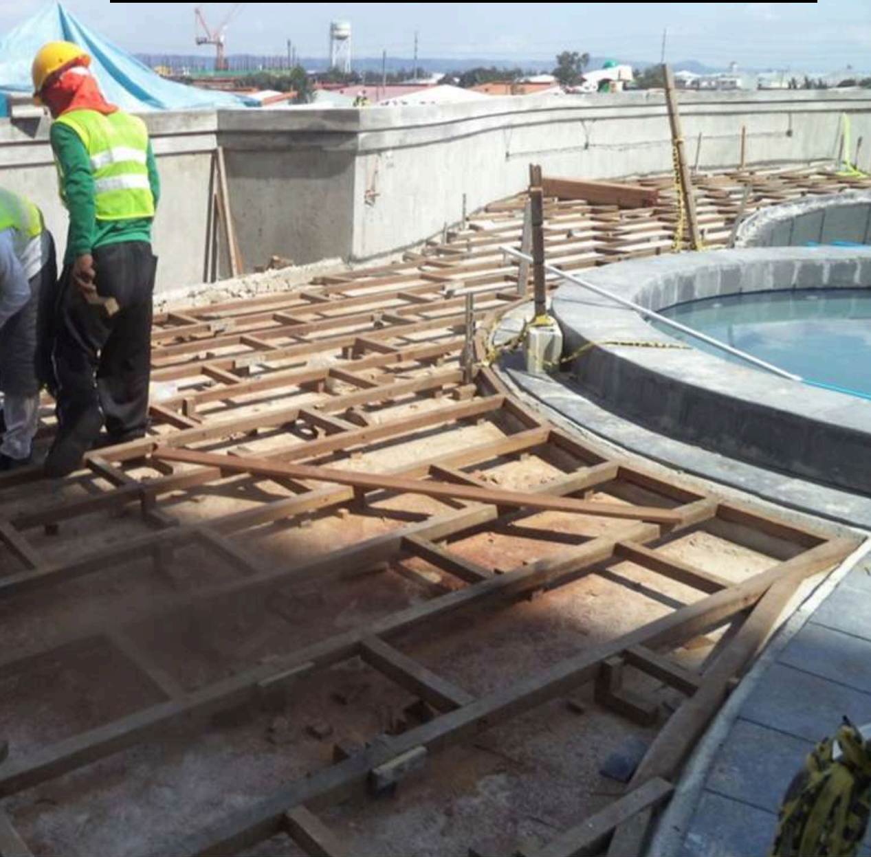
INSTALLATION USING WOOD NAILERS
